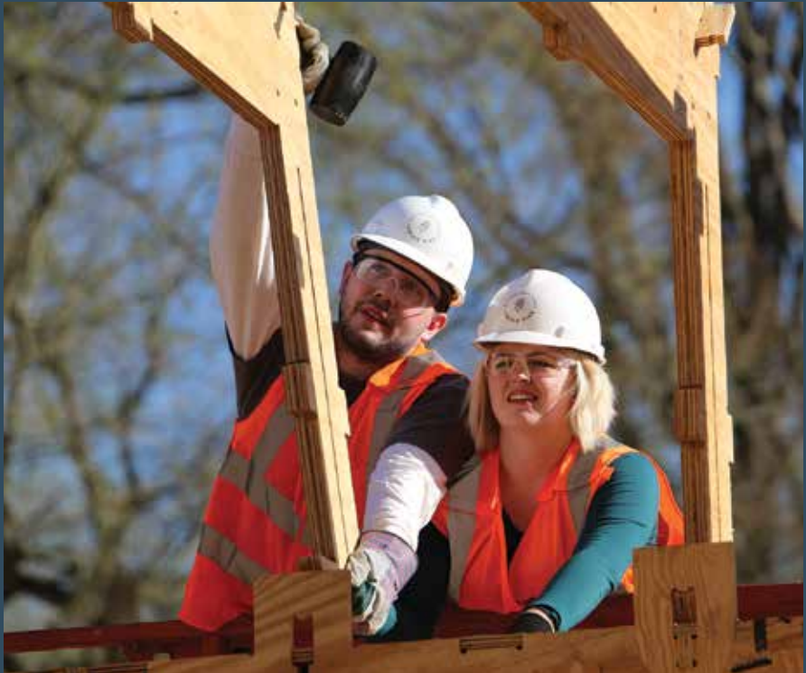
Justin Hamrick lugs a precut section of frame that has been numbered by the CNC machine—a computer-guided router—with its exact place in the structure. Hamrick has put several thousand miles on his truck driving back and forth to suppliers.
